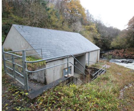
Lowerymore is a "low head project". The Gross head is 18.5m. The pipeline is approx. 175m long by 1.4m diameter made from polyethylene.
