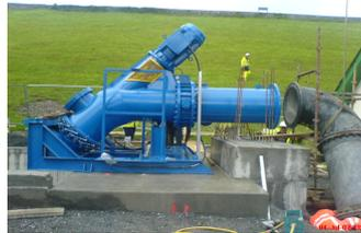
The turbine selected utilises water lubricated bearings to remove the risk of oil / grease contamination of the water. The waterworks at Vartry are of major importance and will at all times take precedence over the turbine operations. A bypass was installed to ensure that water is available to the treatment works at all times. The water turbine operates in parallel with the existing ESB supplies to the waterworks.
